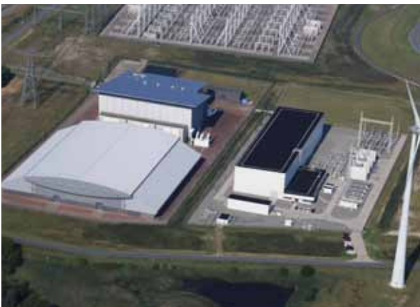
Converter station TenneT | NorNed (left) - undersea high voltage cable between Eemshaven (NL) and Feda (N) and TenneT | COBRA (right) - cable between Eemshaven (NL) and Endrup (DK).
